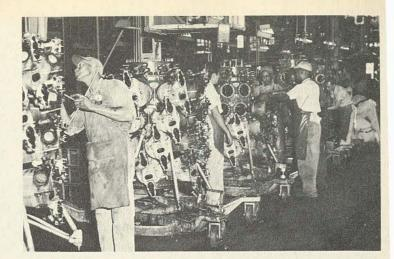
Engine disassembly line
