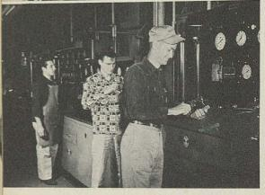
Above: spark plug inspection line, integral oil testing and oil cooler valve test.
