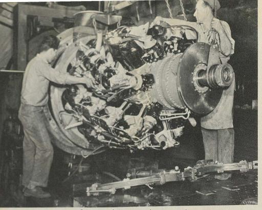
▲ B-36 engine being mounted on test stand
