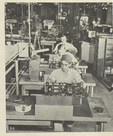
Carburetor repair line in Engine Repair Branch
