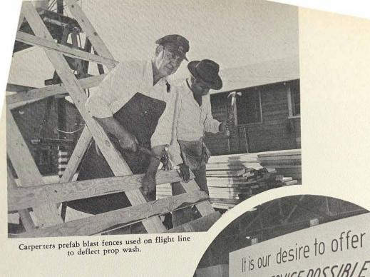
Carperters prefab blast fences used on flight line to deflect prop wash.
