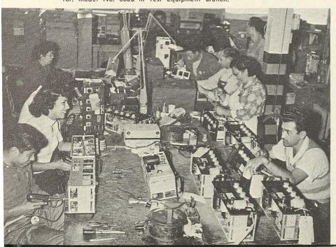
Making up an emergency kit to go with the "Gibson Girl" radio. In the rear is the box kite to carry the antenna, the tall can contains chemical to make hydrogen gas and the small can has the balloon to send the antenna aloft.
