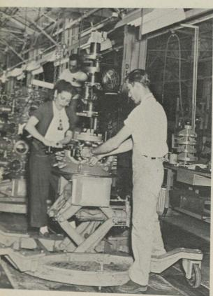
B-36 engine disassembly line
